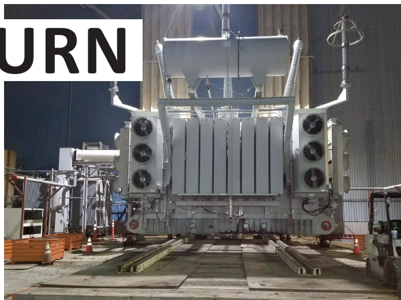
A HT500 skids a failed transformer out of an electric generating facility during a recent emergency operation.
