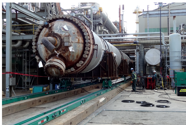
Six JLS250 shoes are connected hydraulically, increasing the total skid system capacity to 900 tons, while maintaining equal load support and weight distribution across all jacking points.
