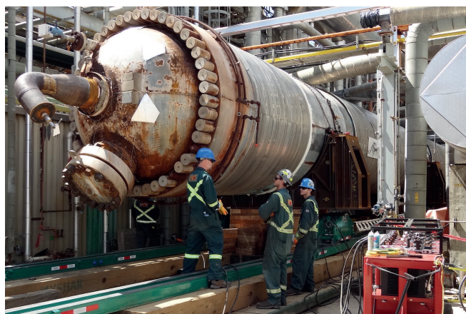
The old converter shell weighed 514,500kg and was 2.7m in diameter and 32m in length. It was jacked up and skidded horizontally in one piece more than 50m.
