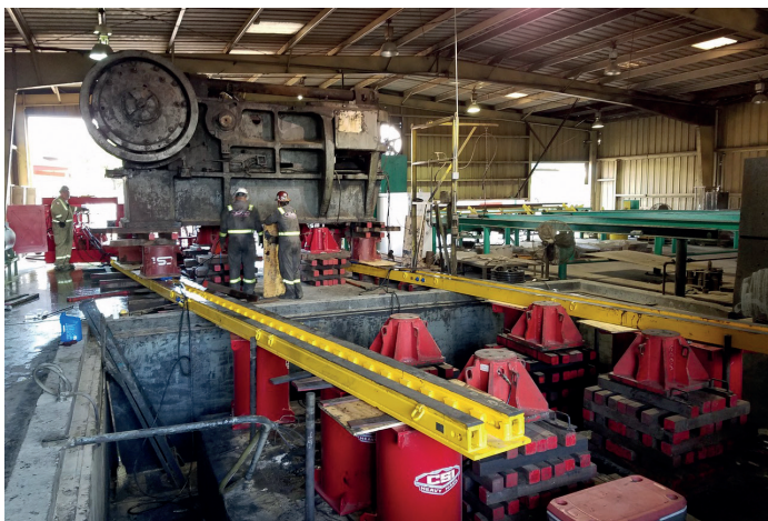
The pipe bending machine is raised 6 ft. out of a pit before being skidded over 60 ft.
